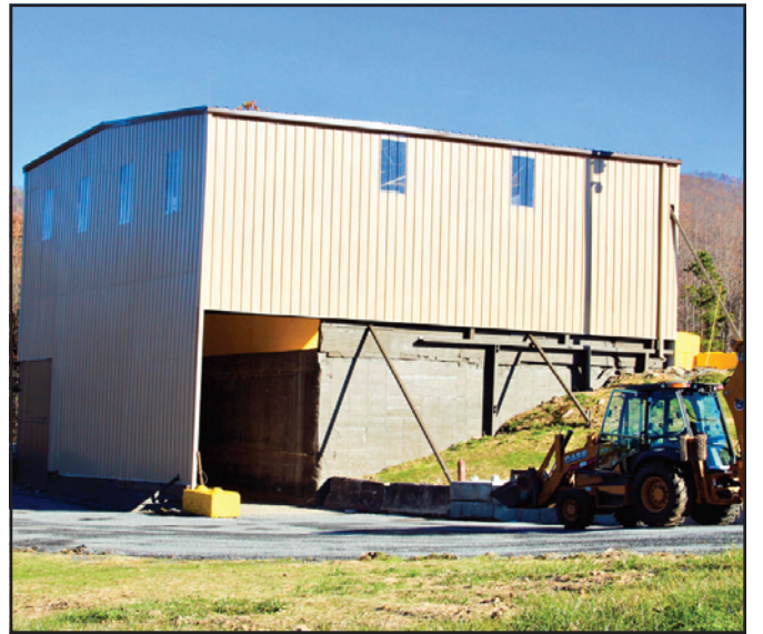
As of Nov. 22, commercial dumping is back in business at the new and improved Union County Transfer Station.
